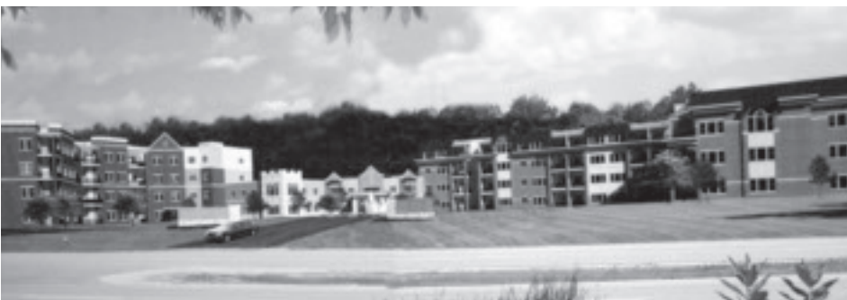
An artist's interpretation of "Sacred Heart at Monastery Lake" located on the original site of Sacred Heart Monastery. Construction is expected to begin by the end of 2009.
